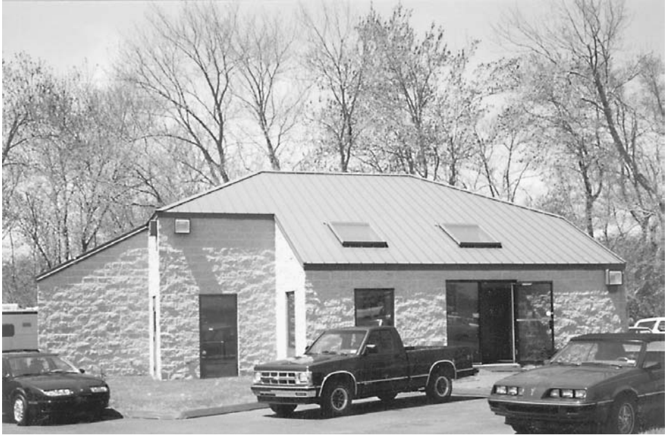
FIGURE 10.1 Despite having a metal roof, this small but complex building with masonry walls would not be an ideal application for metal building systems.
